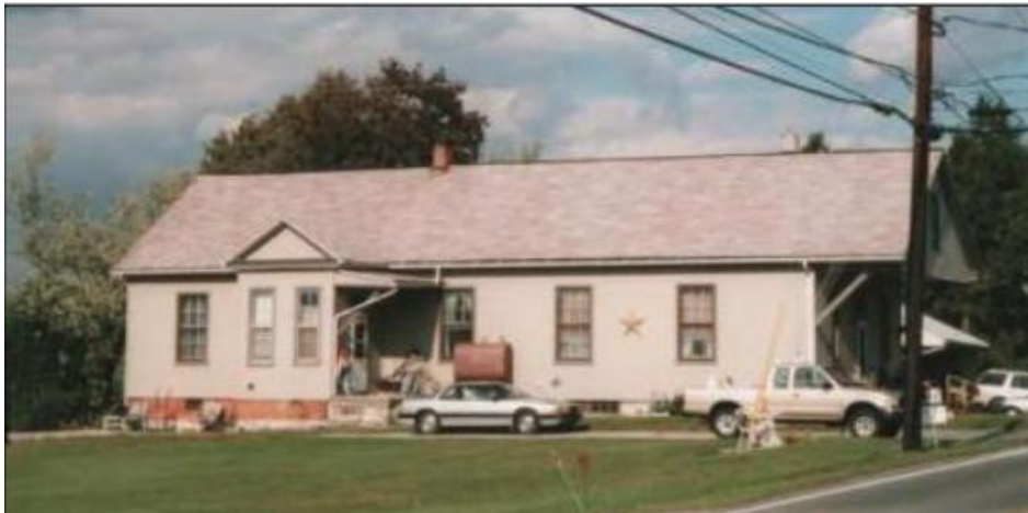
The brick of the earlier section toward the back of the school house can be seen in this photo taken in 2010. Photo by M. Xakellis.
