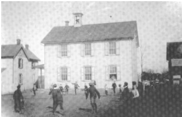
Playground behind Warwick No. 1 Photo courtesy of private collection.
